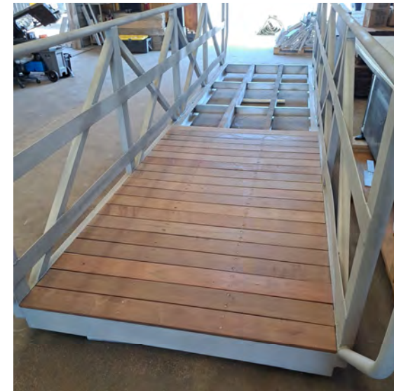
Shown here after blasting and w/50% IPE Deck Boards
