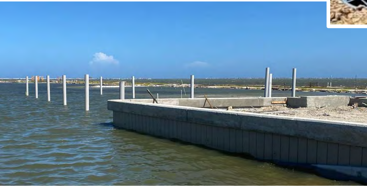
Jetting in the 10ea 12"ECO Pilings Co-extruded Fiber Reinforced PVC (See Center Insert)
