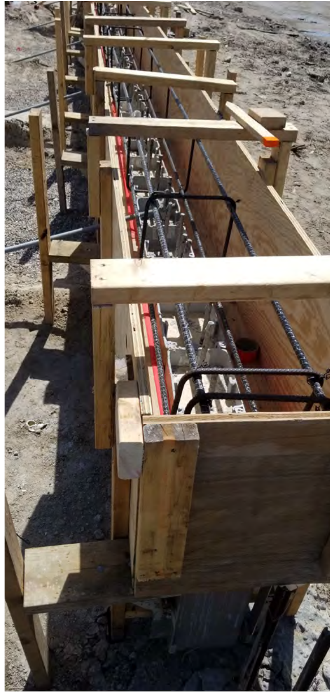
Cap form with basalt rebar
