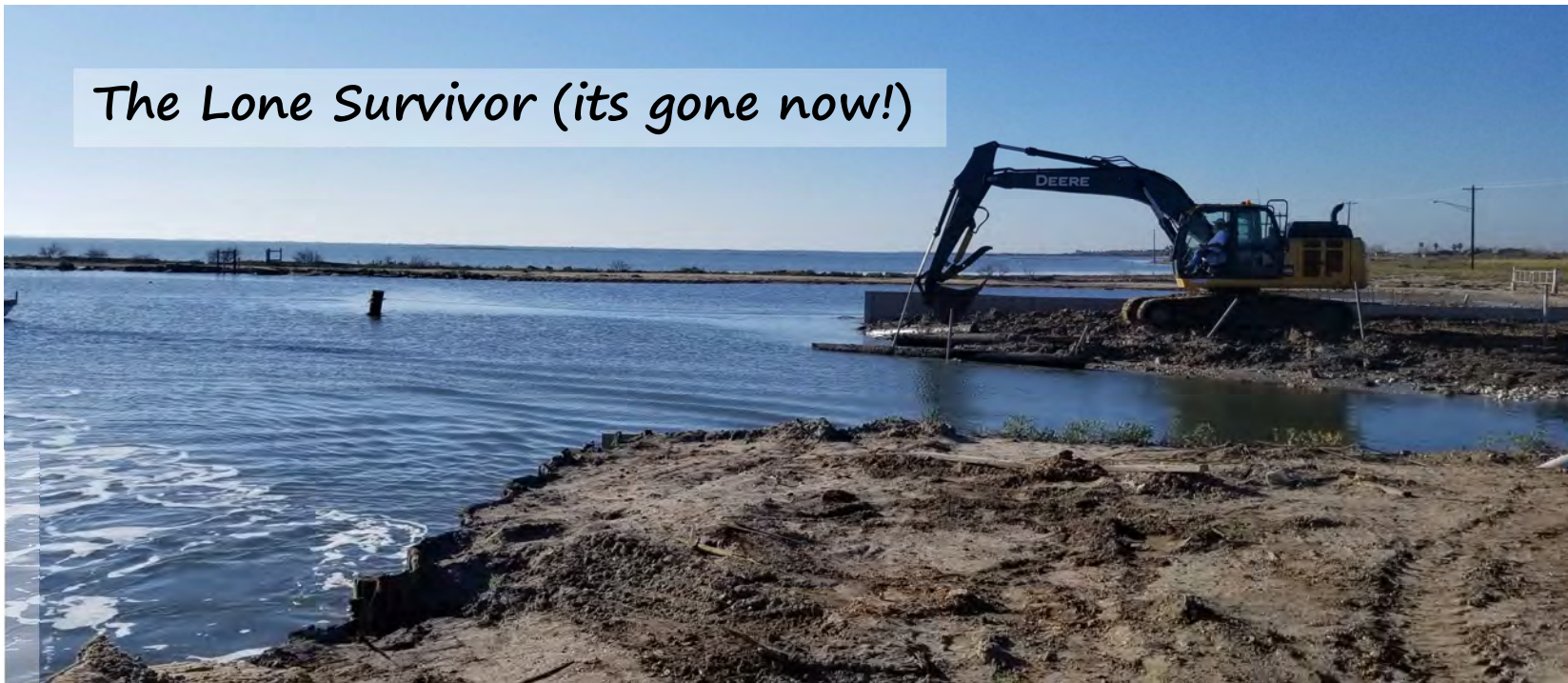
This Crane was a $3000 experiment That was able to pull only 16 pilings or $188/ea, the remaining pilings cost us $300/ea to remove.
