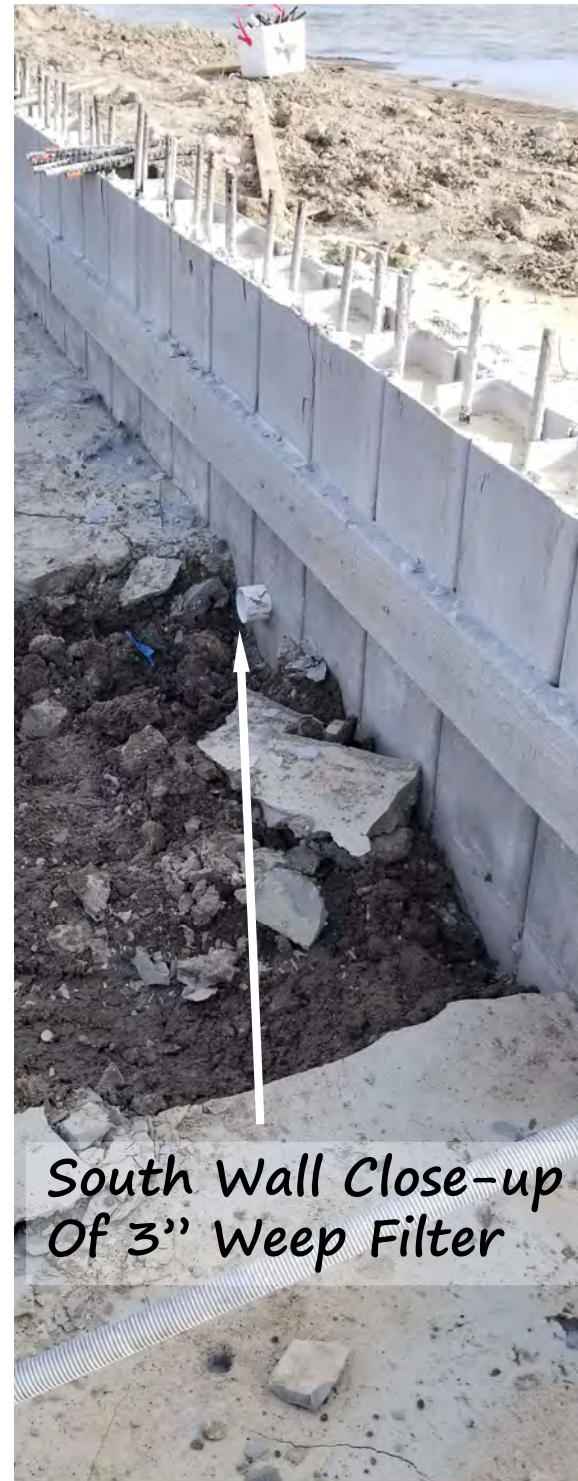
South Wall Close-up Pea Gravel Back Fill for Weep Filters
