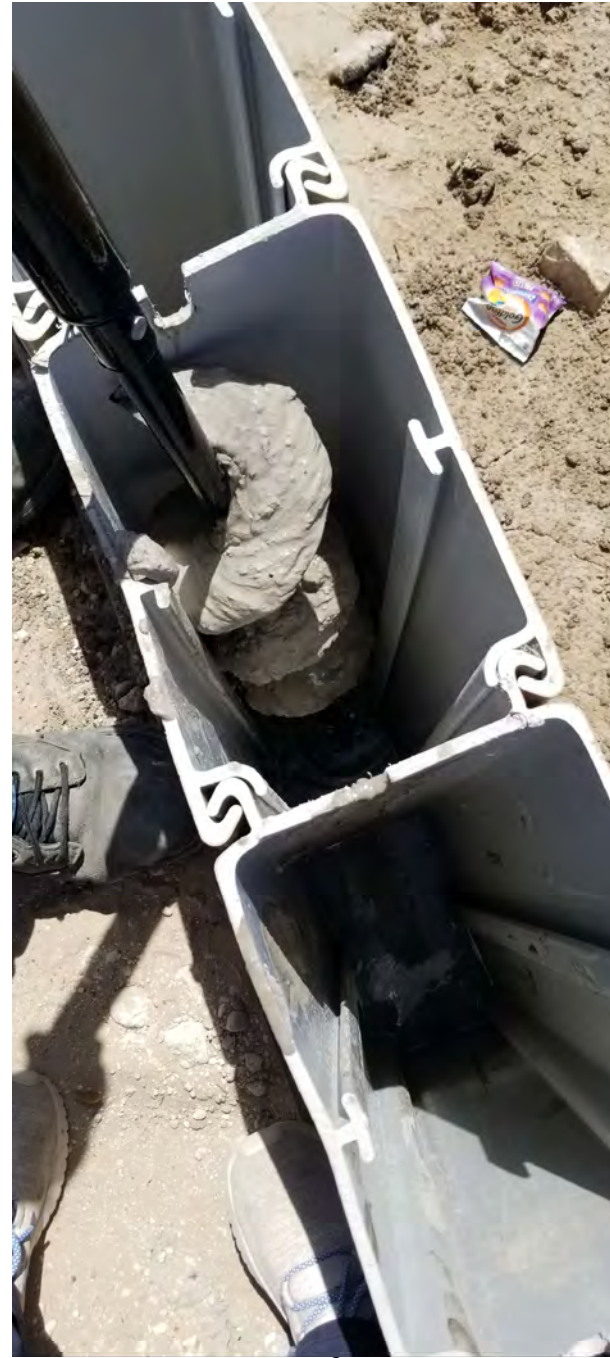
Extraction of mud from each seawall piling
